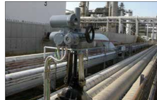
Oil refinery Plant
